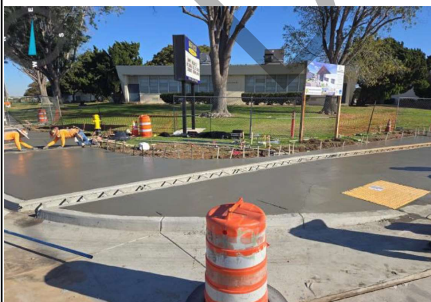
Placing concrete for new sidewalk at NE corner of 17th St and Grove Ave.
